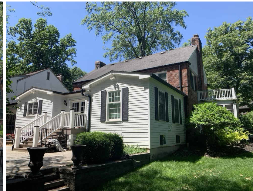
EAST (REAR) FACADE
