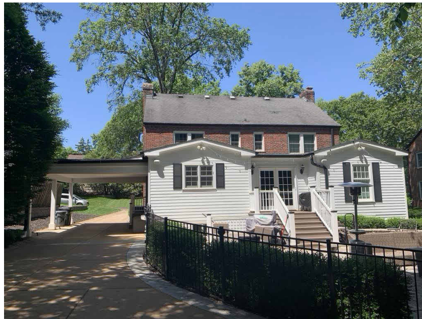
EAST (REAR) FACADE
