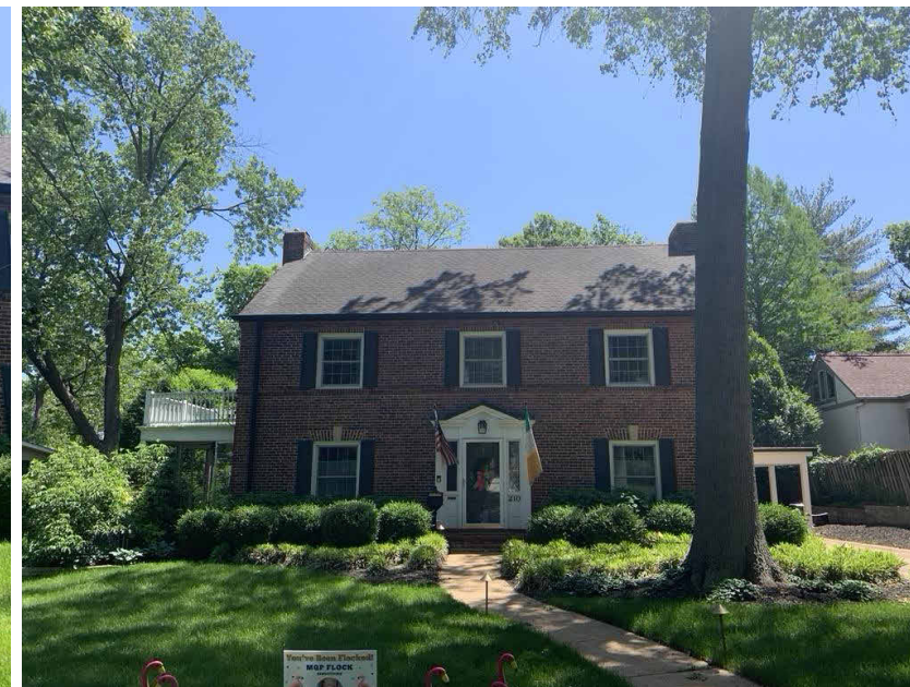
WEST (FRONT) FACADE
